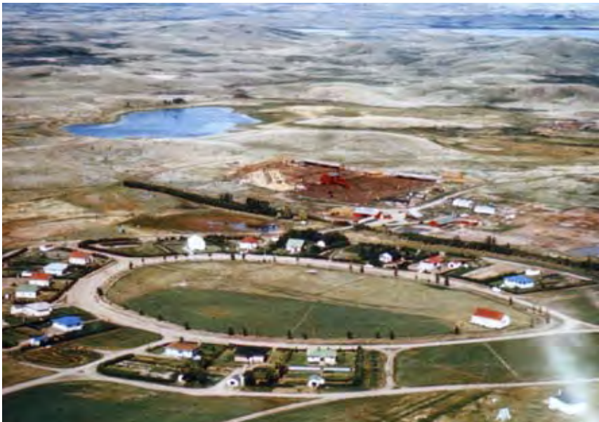
Building site, Matador Co-operative Farm, for its 17 members.
