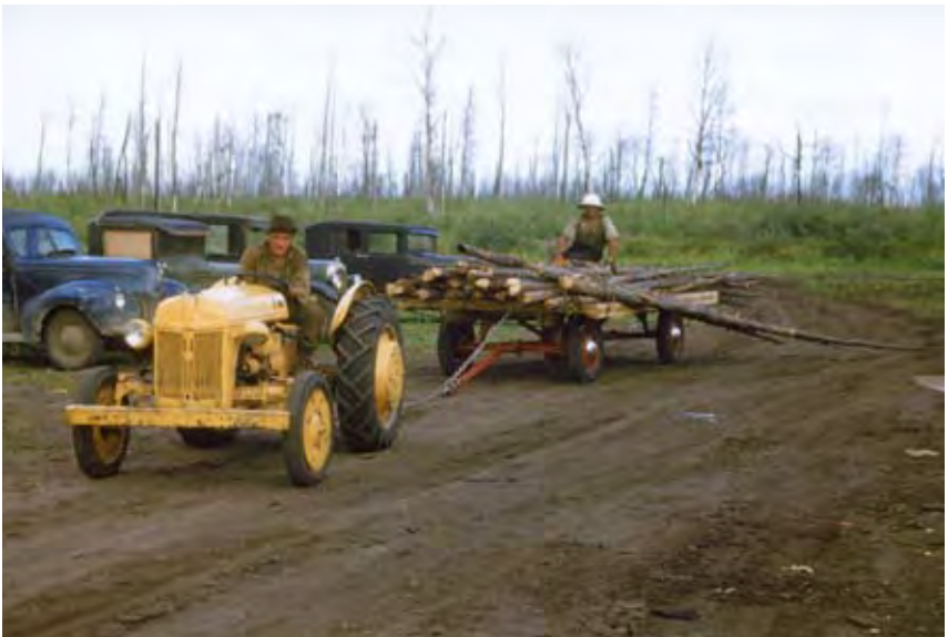
Burnt logs being removed on Carrot River Veterans project.
