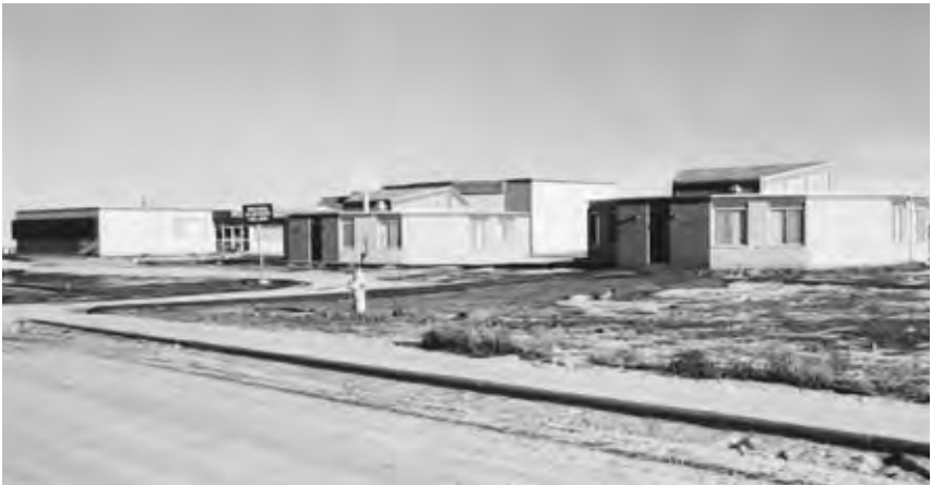
Western Co-operative College building.
