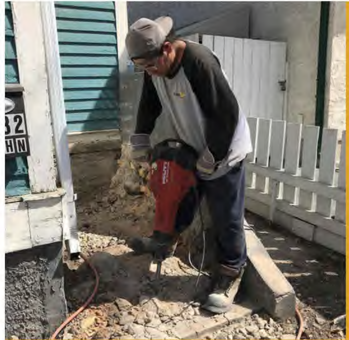
Image 1: Build Up participant demolishing worn concrete steps.
